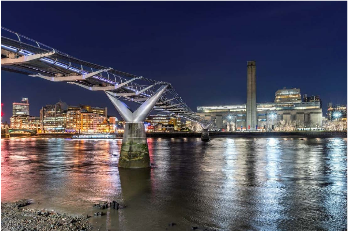
Millennium Bridge – Existing
