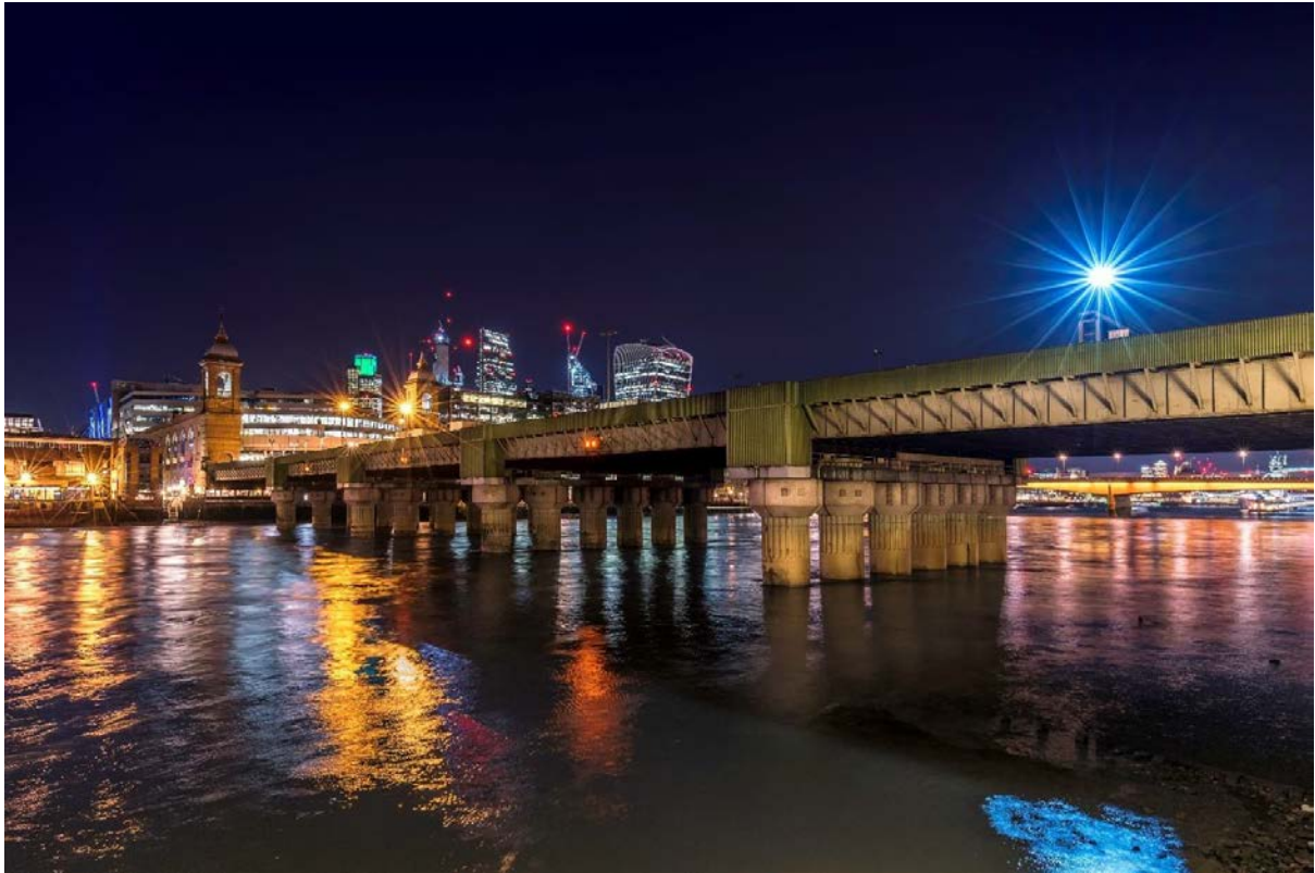
Cannon Street Rail Bridge – Existing
