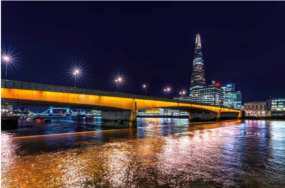
London Bridge – Existing
